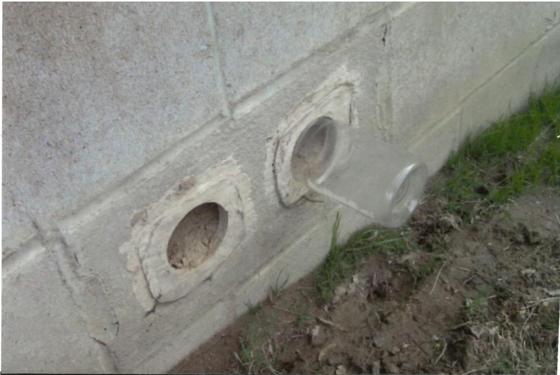
Figure 4. A photo of Block 5 in the North Lot Retaining Wall. Note the trap jar inserted into the 5E aperture (right) whereas the 5W aperture (left) is open to the environment.
