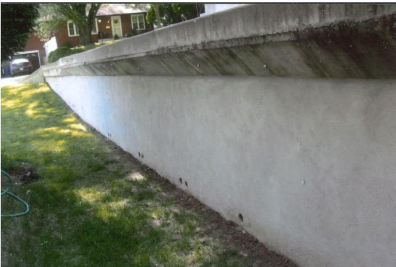
Figure 5. A photo of a portion of the North Lot Line Retaining Wall looking west after the wall had been plastered over in June 2018.
