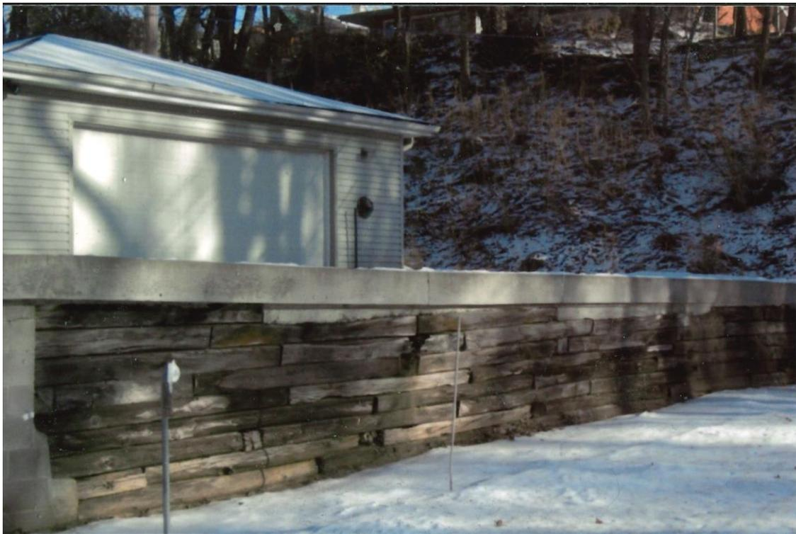
Figure 2. The railroad tie portion of the North Lot Retaining Wall, 3624 Virginia St., Sioux City, Iowa, This photo taken in winter 2013.
