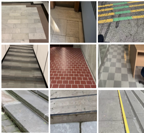
Figure 3. Examples of incorrect environment predictions by the convolutional neural network. The first row contains level ground images that were misclassified as level ground – incline stairs (LG-IS). The second row contains level ground images that were misclassified as incline stairs (IS). The third row contains images from the stair classes that were misclassified as level ground (LG).
