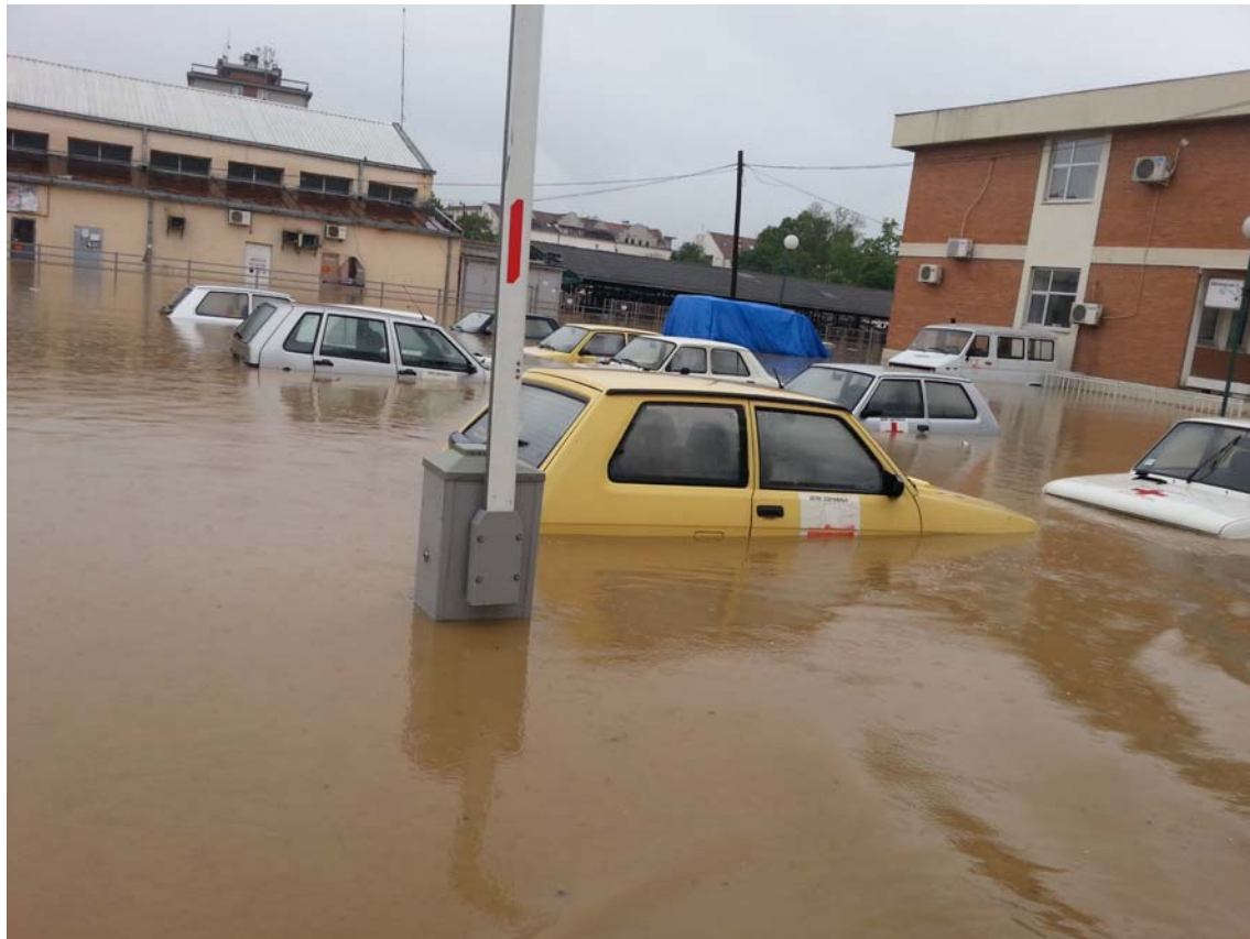
Figure 2. The flooded parking lot and Primary Healthcare Centre's building during the floods of 2014.
